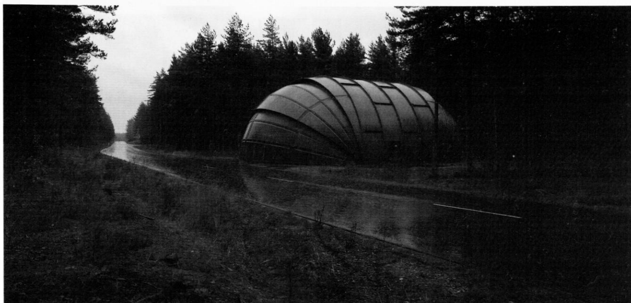
Above and Below - The Unique aircraft shelters, on the taxiways at Eskilstuna - Photo By Mark Bennett
